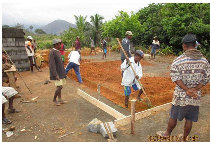
Figure 21: Digging the foundations for the Ambodilazabe Primary School.
