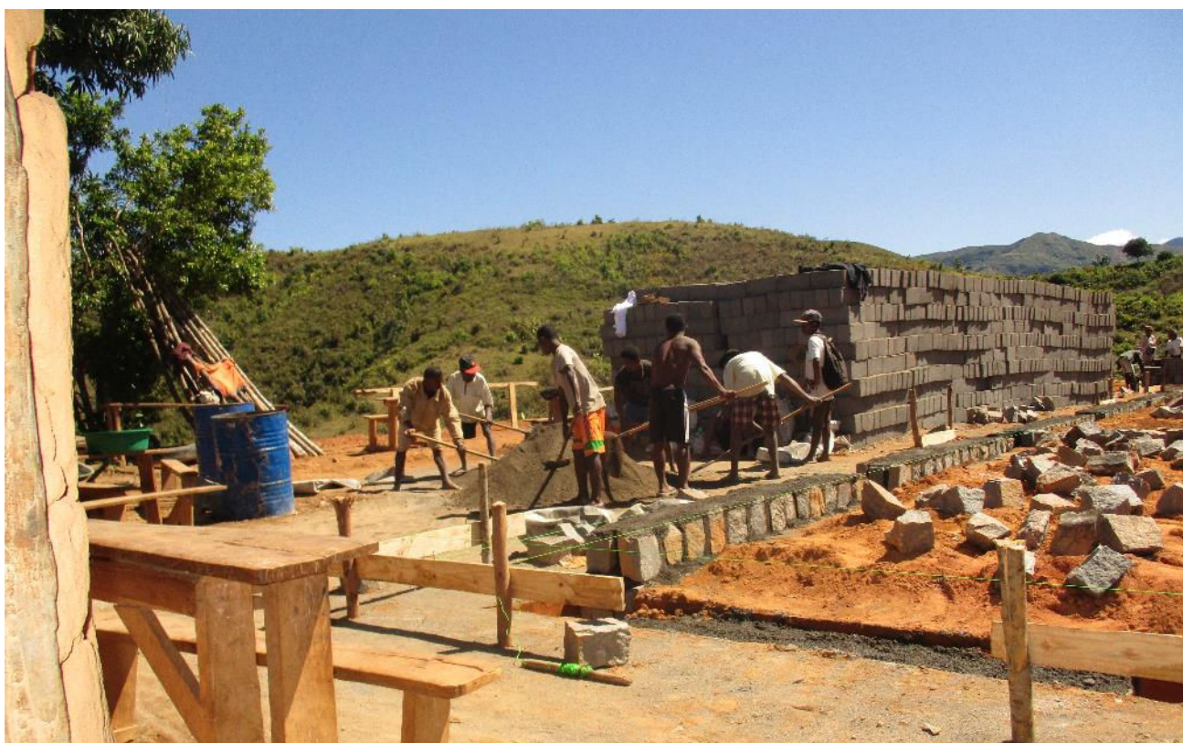
Figure 18: Laying the foundations for the new Ambodilazabe Primary School.
