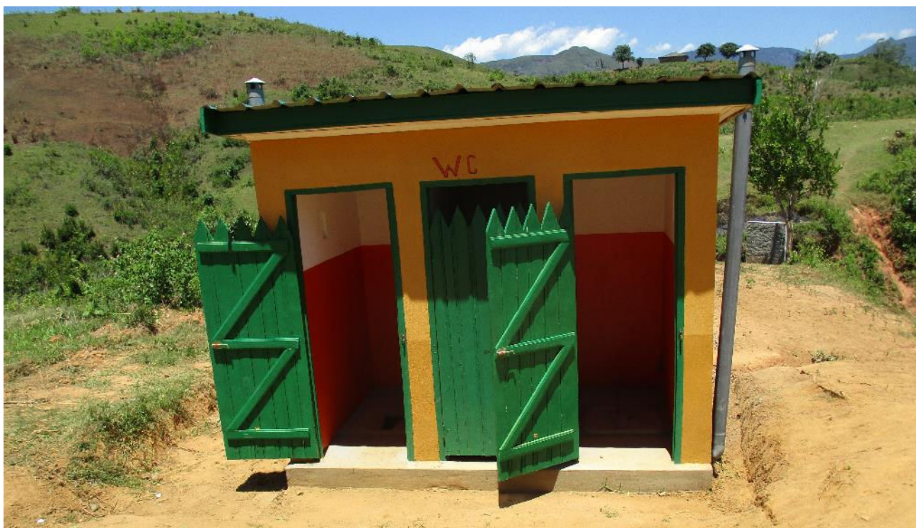
Figure 7: The 'fly-proof' latrine compartments.
