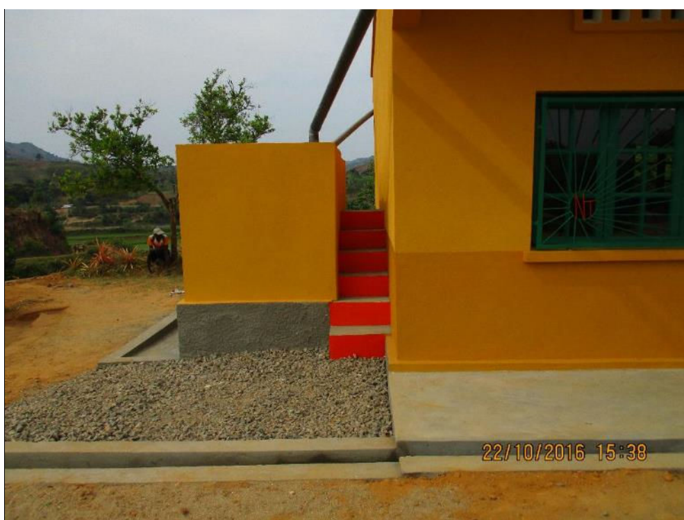
Figure 8: Steps leading up to the impluvium tank in order to refill during dry spells, or to clean inside.
