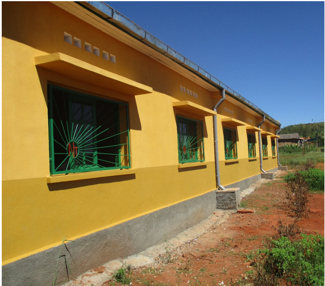
Figure 14: Posterior view of the Teloambinifolo Primary School with protection for the down-pipes.
