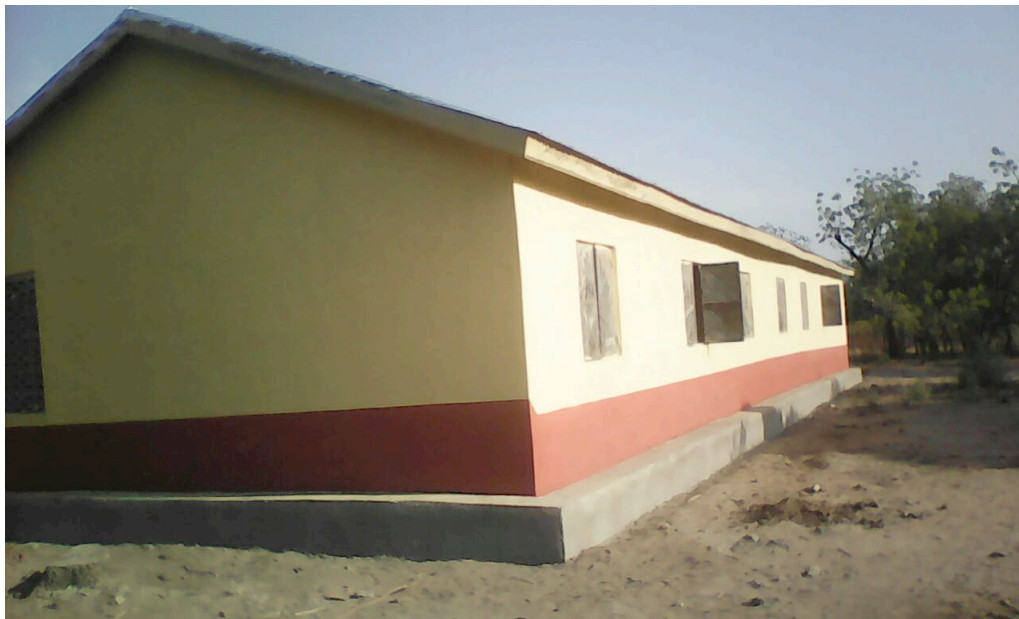
Rear of the school showing the reinforced apron which protects the foundation and walls from erosion
