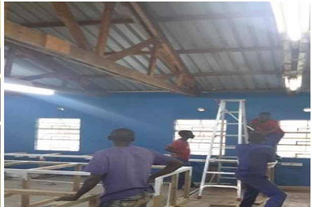
Refurbishment of classroom
