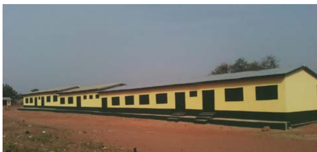
The completed reroofing of Naa-Sheriga Primary School. December 20
