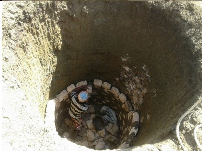
Ongoing excavations of the Dzanekekeni community well.
