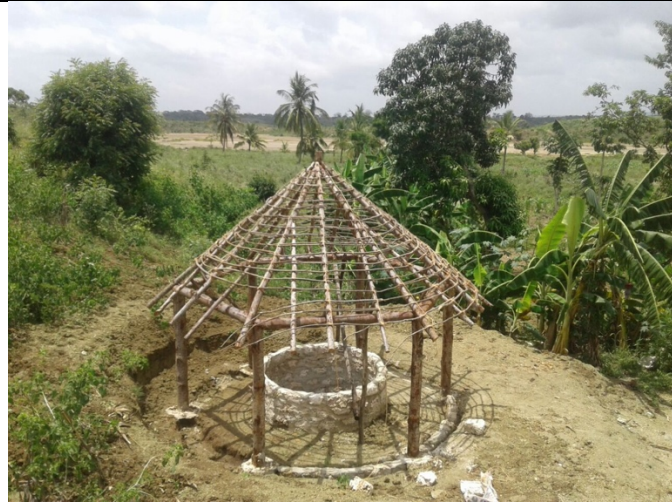
Construction on the roof of the well at Jitegemee.
