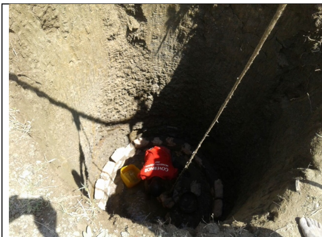
Ongoing well excavation work at the Ufanisi community (depth of 10ft).
