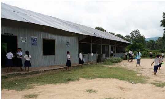
Old primary school building at Domnakorkos.
