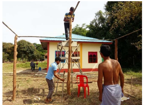
Construction of a teachers house through community members.
