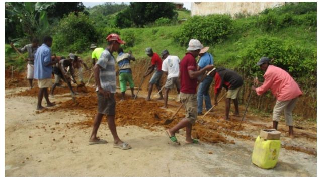
Digging the foundations of the school building.
