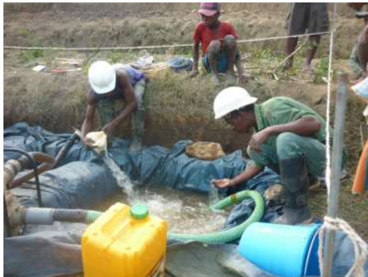
Drilling using the rota jetting technology (adding polymer).
