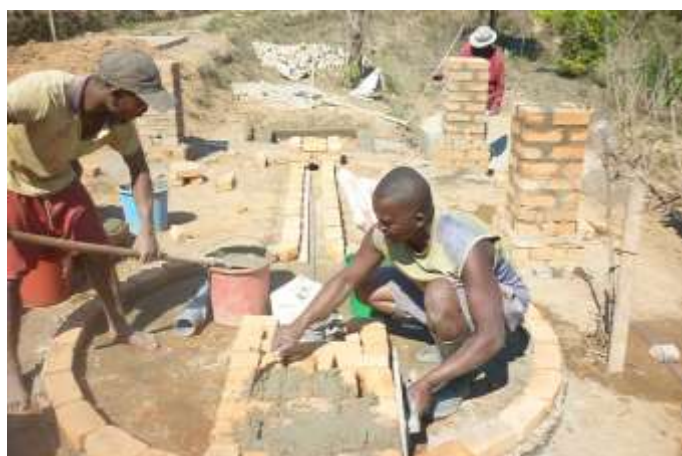
Building the surface structure: a concrete pedestal, sanitary apron, a soakaway ('sump') and a painted fence. The fence serves to prevent animals from entering the well area.
