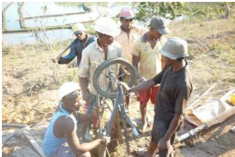
Borehole development using a rope-pump. This was alternated with use of the moto-pump.
