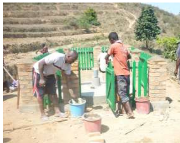
Building the surface structure: a concrete pedestal, sanitary apron, a soakaway ('sump') and a painted fence. The fence serves to prevent animals from entering the well area.
