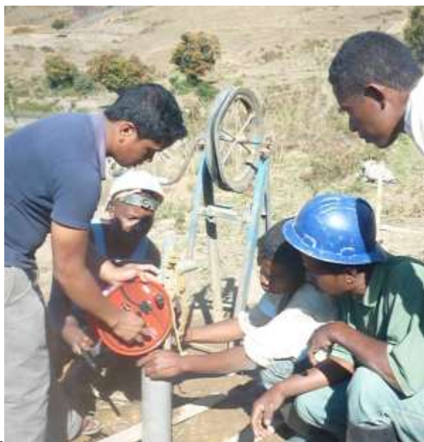
Measuring the depth of the borehole (left) & beneficiaries carrying materials to site (right).
