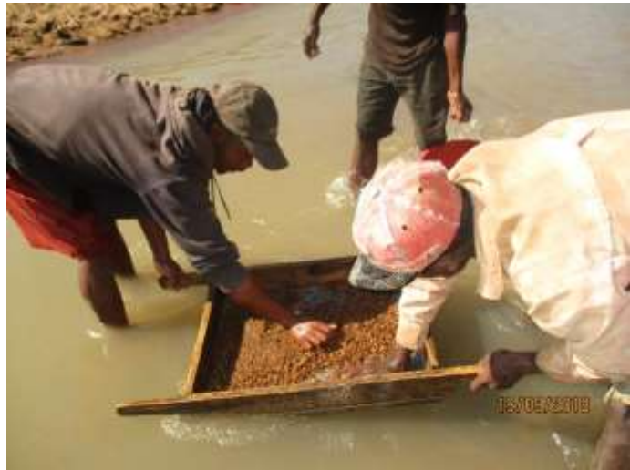
Preparation of the sand filter pack, which was placed in the open space surrounding the well casing.
