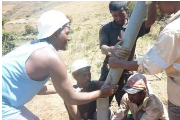
Inserting the PVC well casing.
