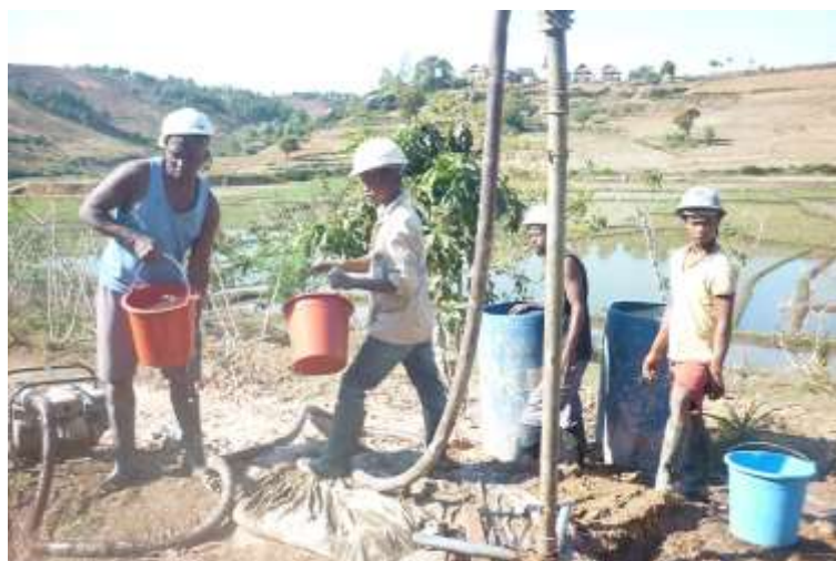
Drilling using the rota jetting technology (adding polymer).
