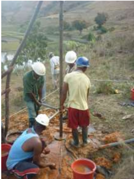
Preparation of the sand filter pack, which was placed in the open space surrounding the well casing.
