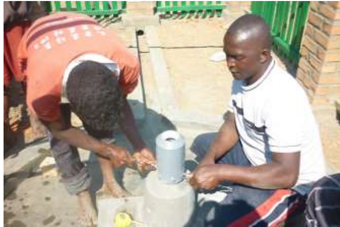
Installing the Canzee hand-pump on the borehole.
