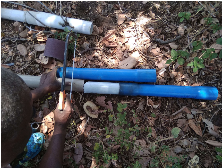
Repairing a broken riser pipe (Mkokwani pump, Kwale county repaired March 2019)
