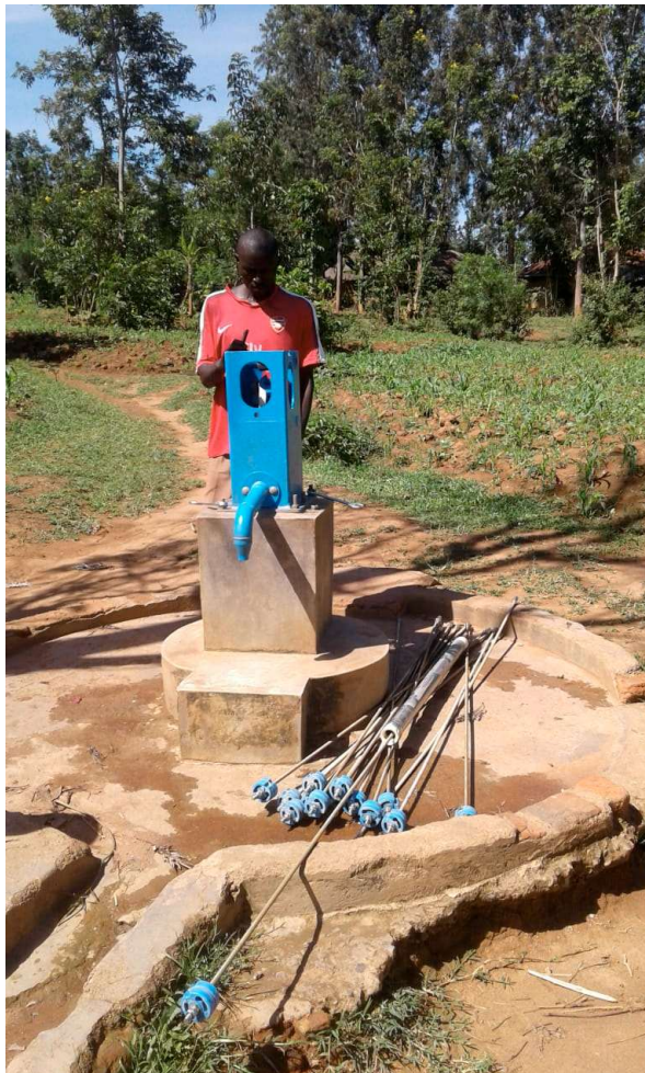
Installing a new pump at Umaje
