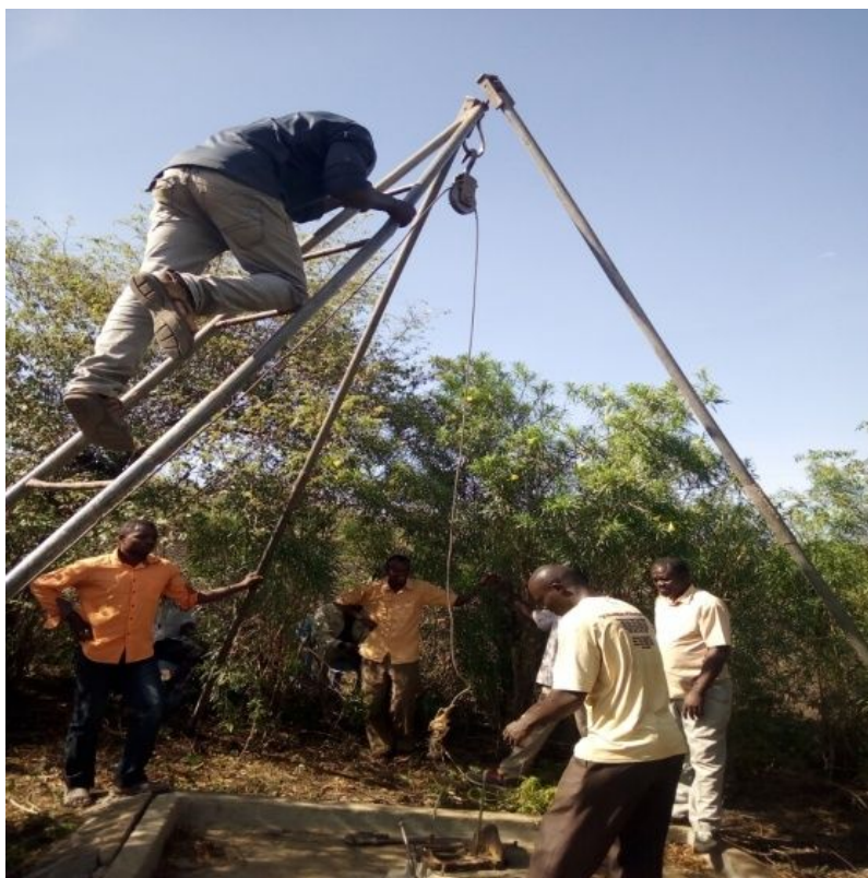
Pump repair 72 - going fishing trying to remove broken pipes. This repair is still ongoing.
