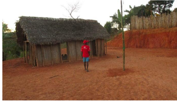
Figure 2 : The building site already levelled and ready for building.
