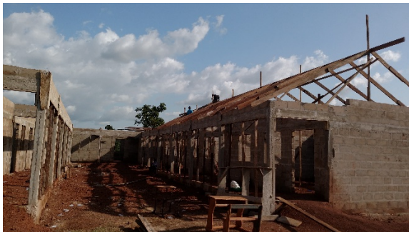
Adding the eaves and the zinc covered roofing panels.
