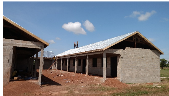
Adding the eaves and the zinc covered roofing panels.
