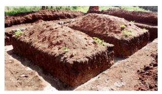
At Kachere, pictured below, foundations have been constructed and the structure is ready for its concrete base to be built.
