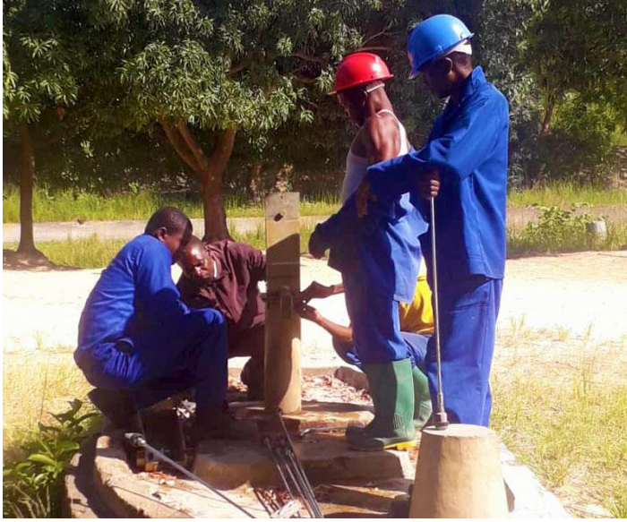
Repairs being carried out to a borehole in Nkhata Bay District
