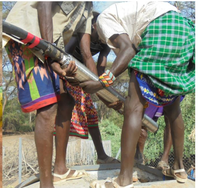
The big new pumping unit being put back in the borehole
