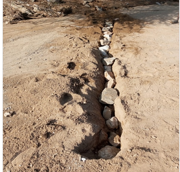
Covering the pipe with a solid foundation
