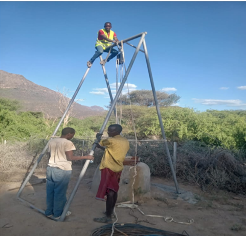
Removing the pump
