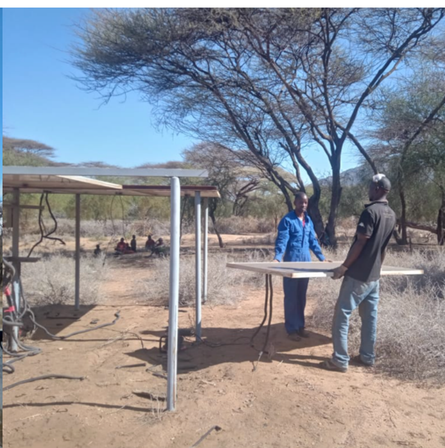
Moving panels from the old system to the new
