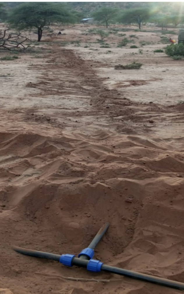
Burying the final sections of pipeline
