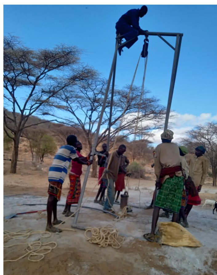
Lowering the new pump into place
