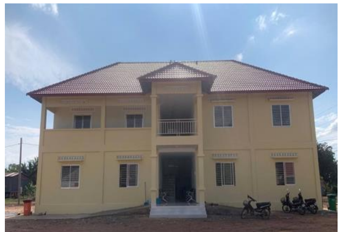
The new Eagle-funded hospital building at O'Chrov Referral Hospital
