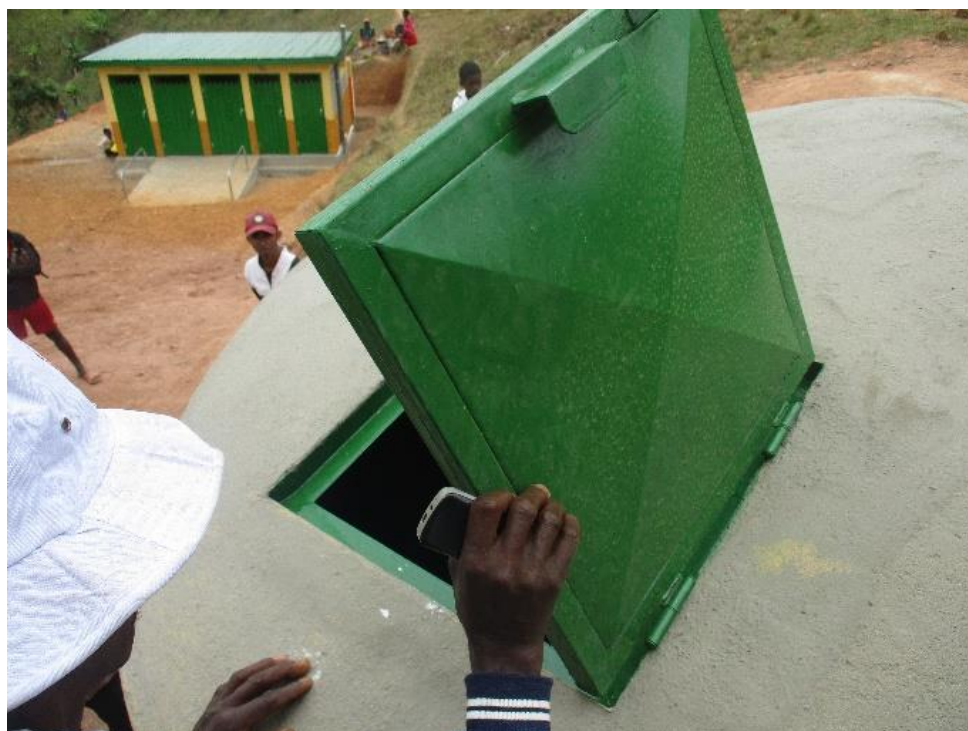
Figure 10 Man-hole lid to the Impluvium rainwater tank
