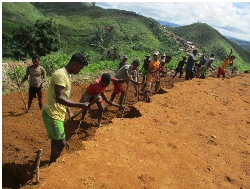
Figure 11 Land levelling in preparation for the support wall construction.
