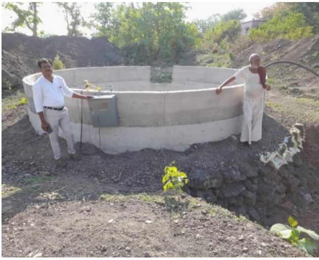
The completed well at Vetawadi Village
