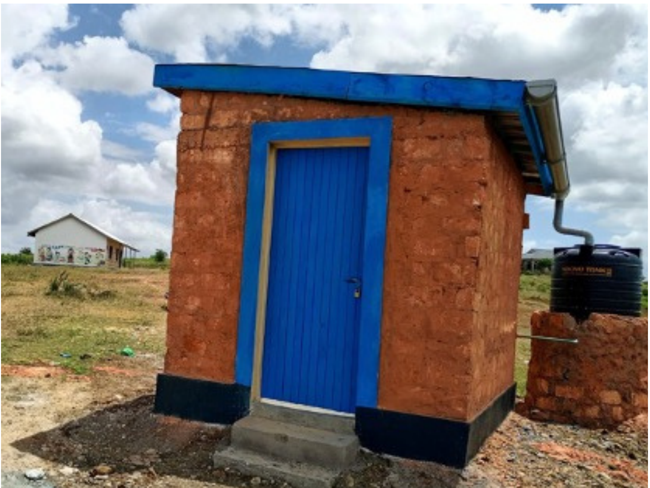
-The completed eco-loo
