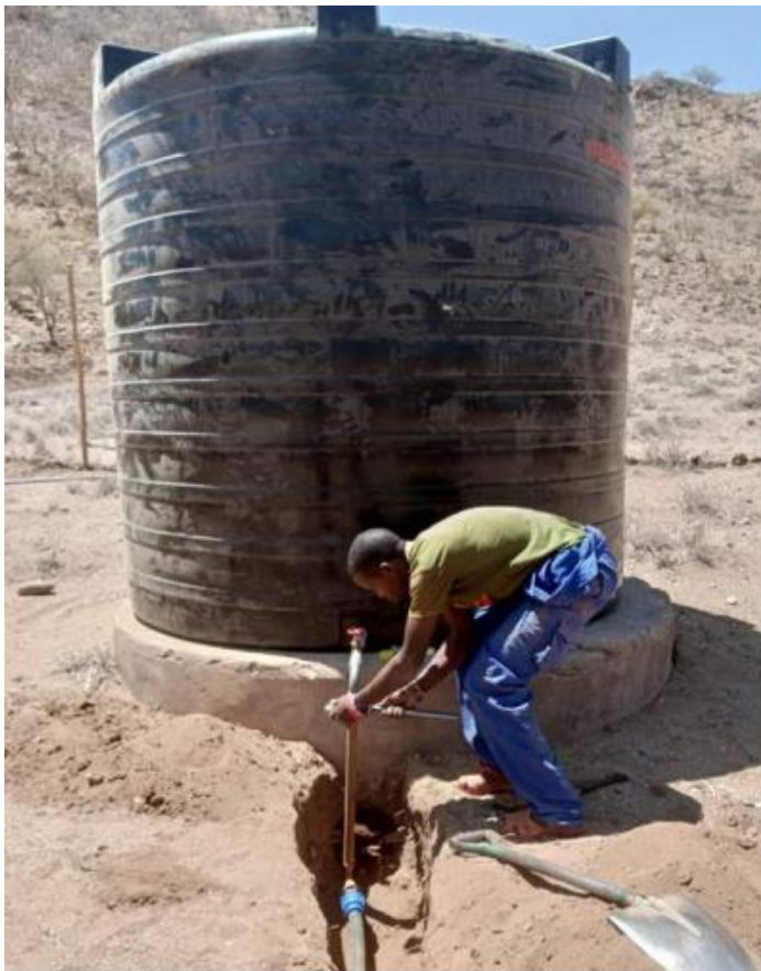
Muko installing the new tank
