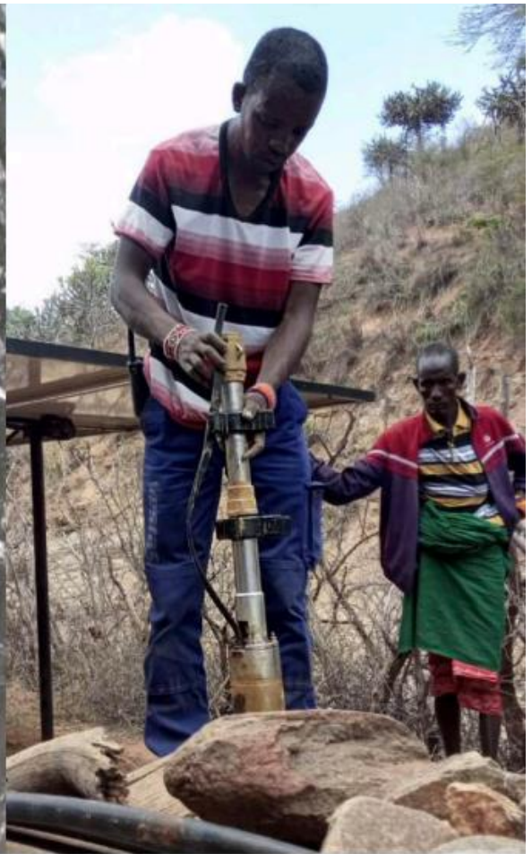
Muko removing the pump for inspection
