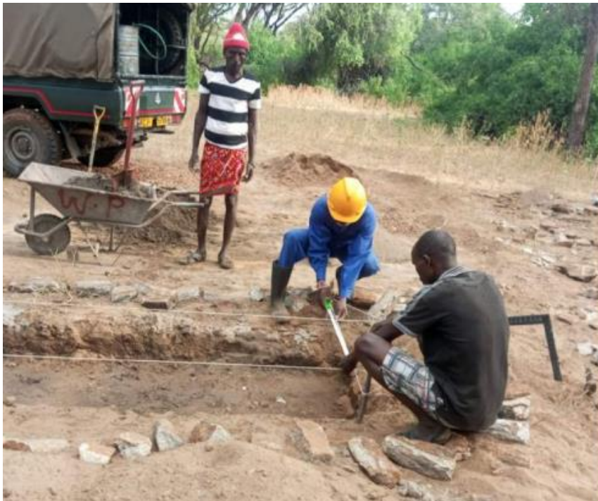
Leveling being done for the new trough
