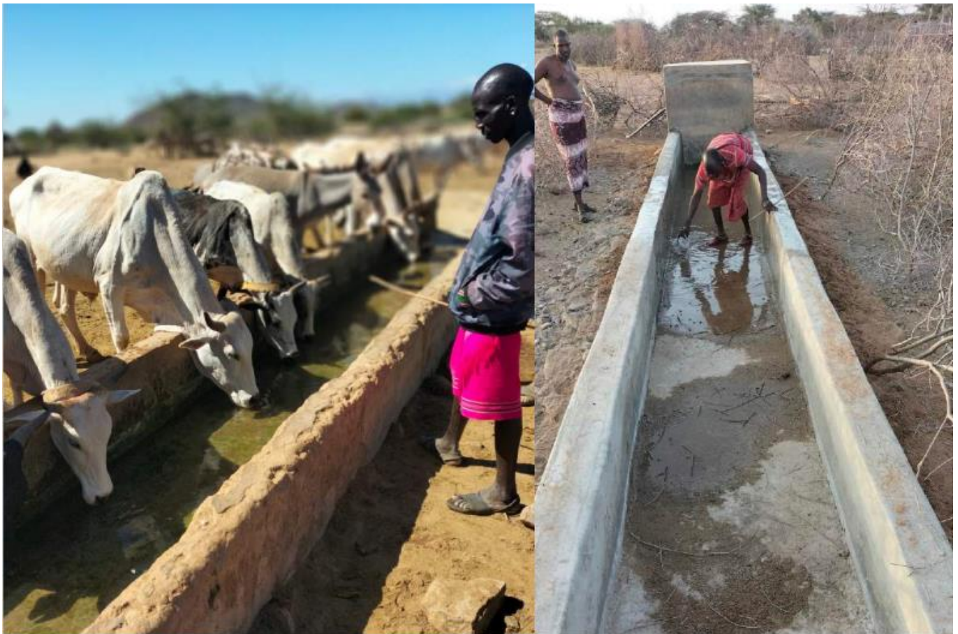
The original trough, showing serious damage
