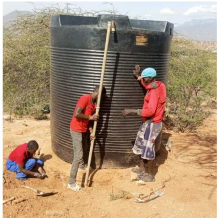
Fitting the new tank from the school
