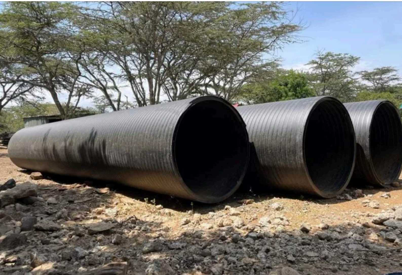
Heavy Duty PVC well linings delivered to site.
