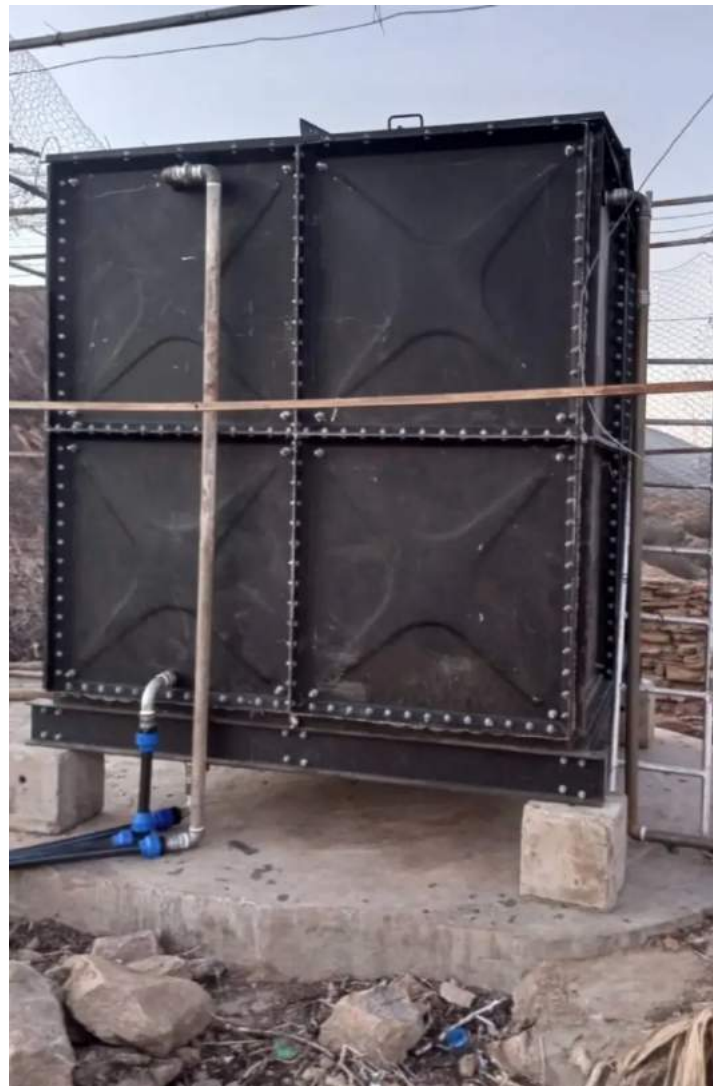
The tank prior to painting
