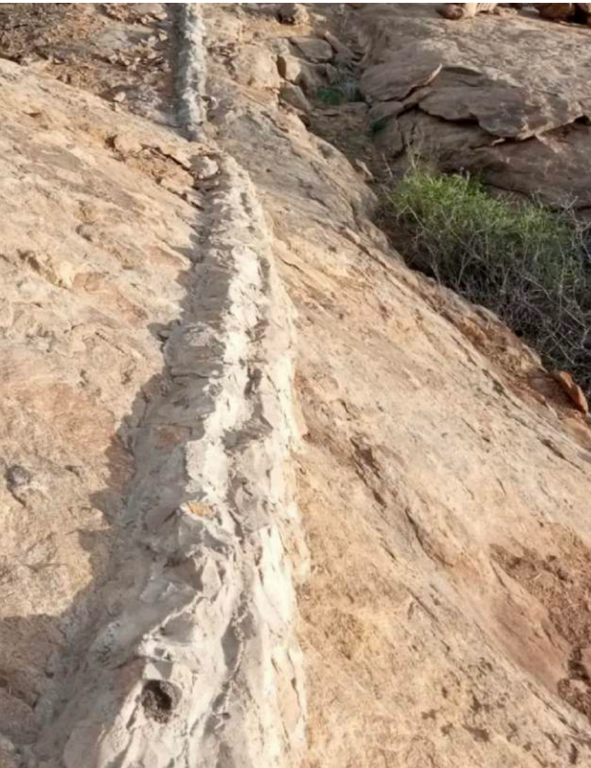
'Elephant Proofing' the pipelines over rocky sections
