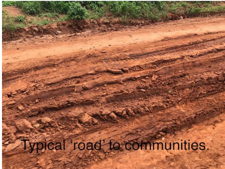
Access road to a rural pump repair
