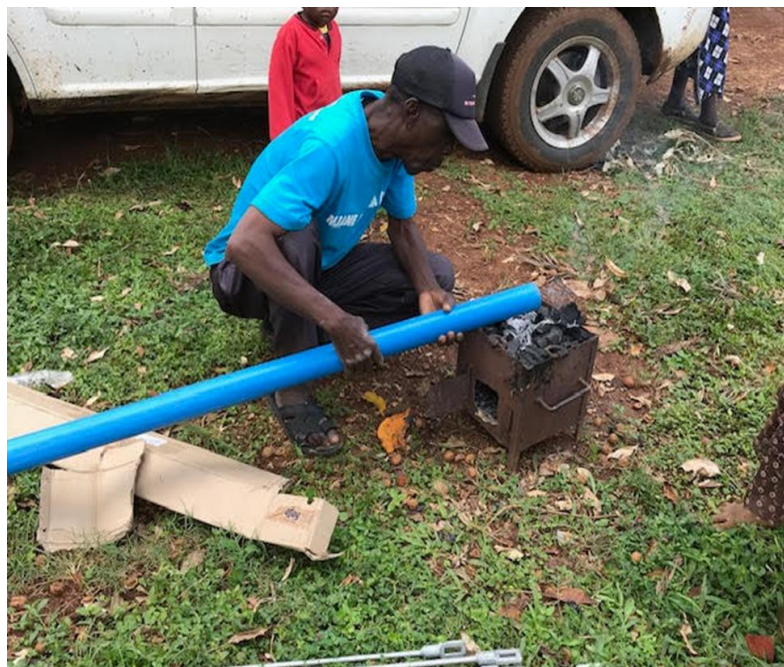
Making a joint to fit a riser.
