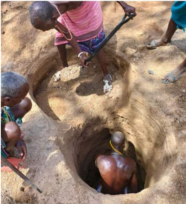
The community digging a deep well
