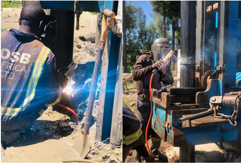
Technicians welding the casings
