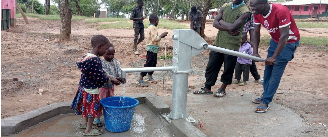
Children enjoying water from the newly constructed well at Biketi school
