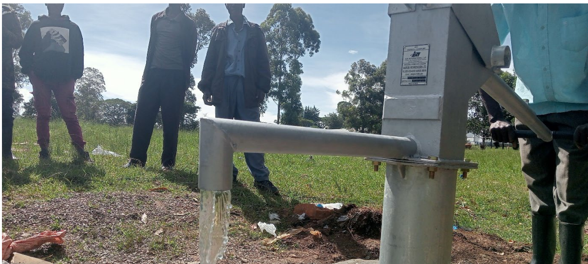
The last stages of installation at Munyaka Primary
