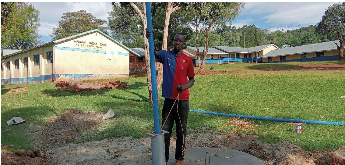
Pump installation at the newly constructed well - Kapsirowa Primary School
