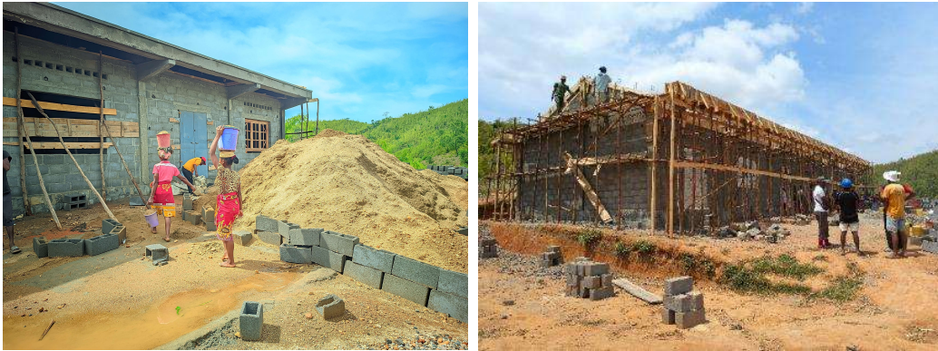
Figure 5: Work in progress
