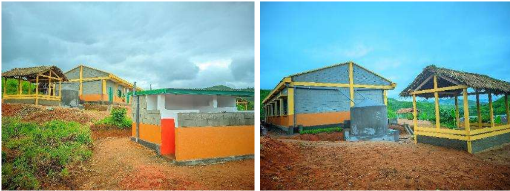
Figure 6: End of the work
