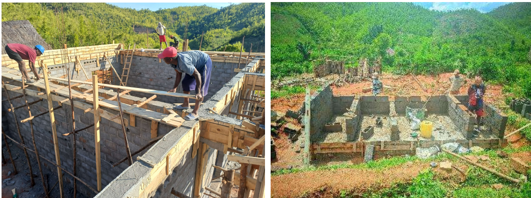
Figure 3: Work in progress
