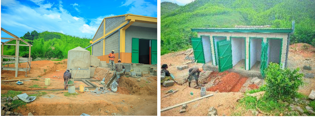
Figure 4: Construction of latrines and impluvium
