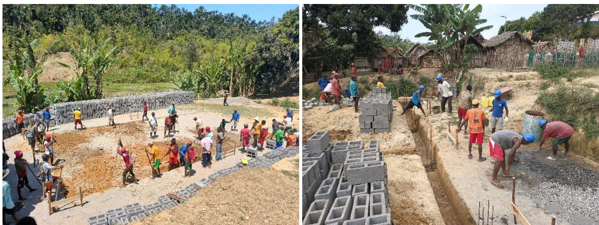
Figure 7 Launch of works (digging and laying the foundations)
