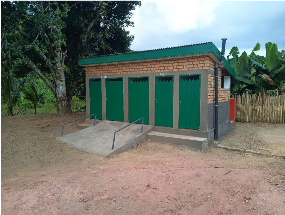
Figure 11 The school sanitary block
