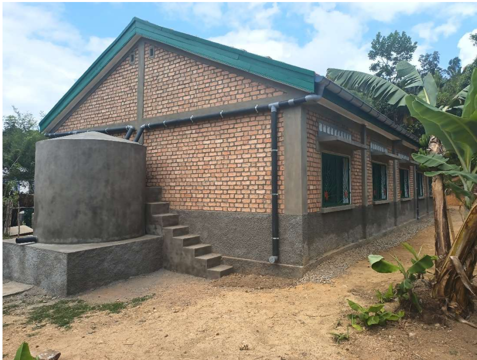
Figure 10 Implusium rainwater collection tank linked to hand-washing facilities.
