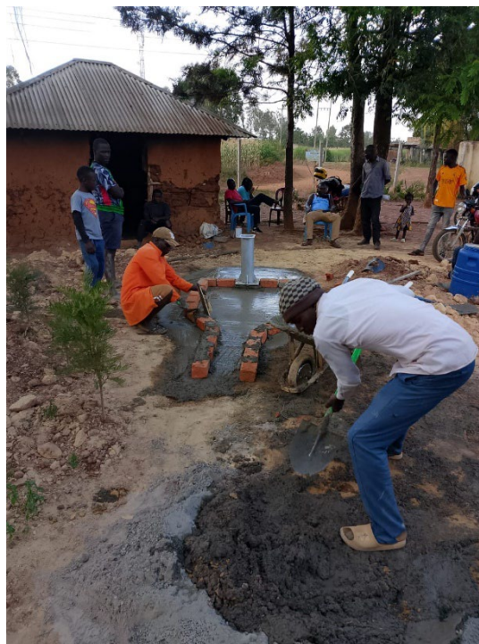
Completing the pad for the well at Nasira Primary
