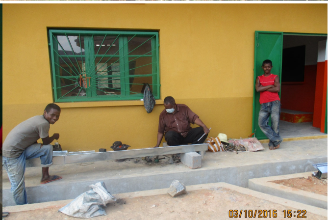
Figure 16: Installation of guttering at Tanakambana Secondary School.
