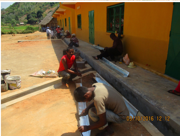
Figure 16: Installation of guttering at Tanakambana Secondary School.
