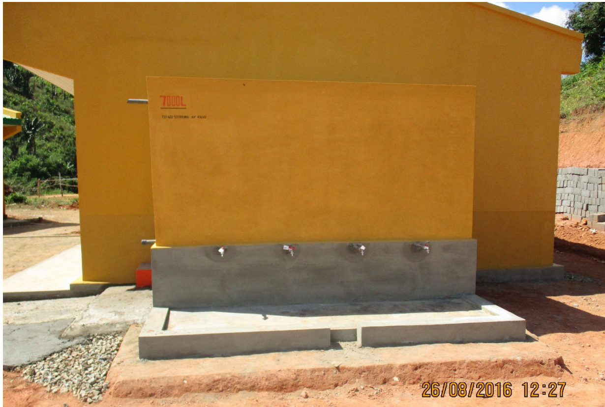
Figure 5: The water tank and hand-washing station (before installation of guttering/down-pipes).
