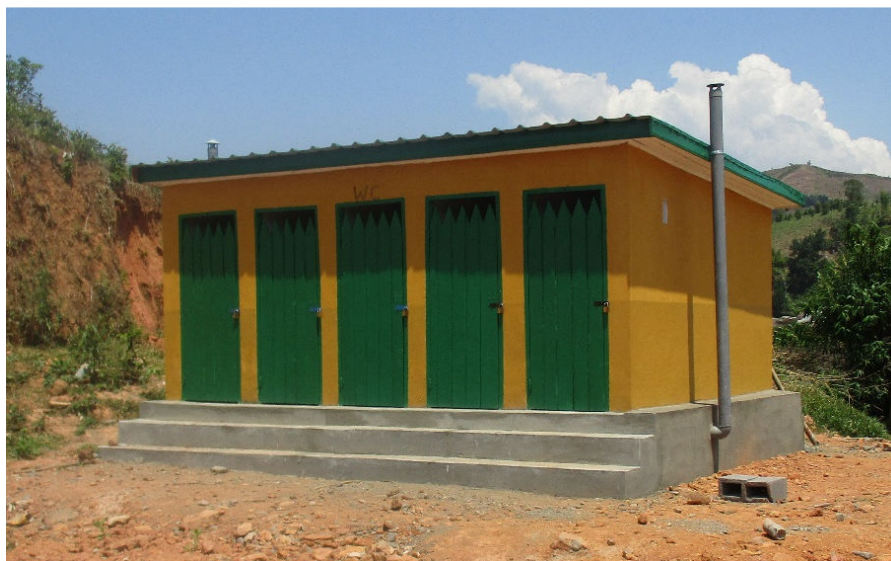
Figure 6: The 5-cubicle sanitation block.
