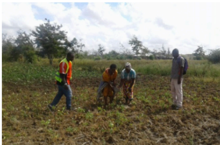
14.10.2016: ESF site is pegged
