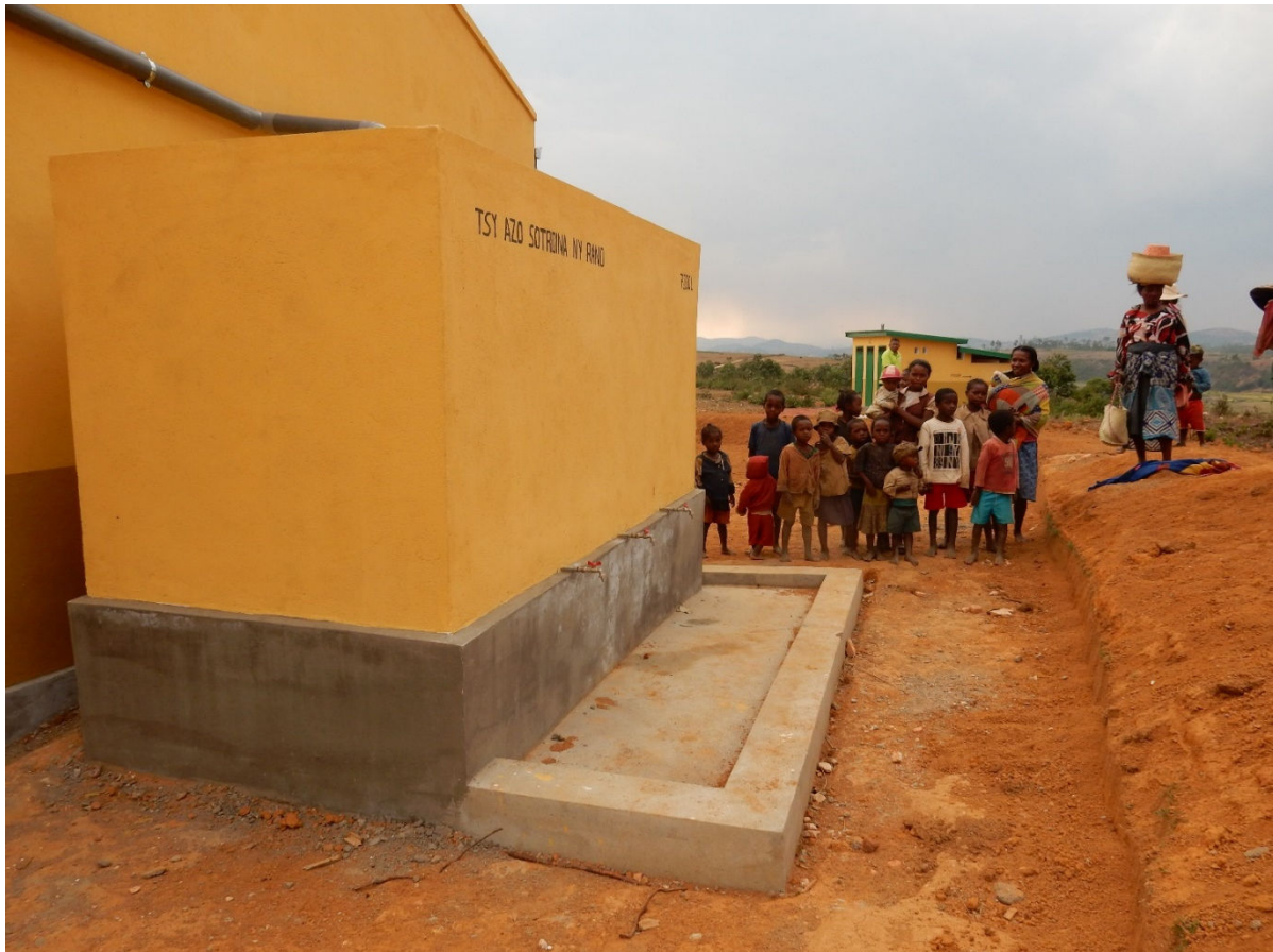
Figure 9: The 'impluvium' rainwater catchment tank & hand-washing station.
