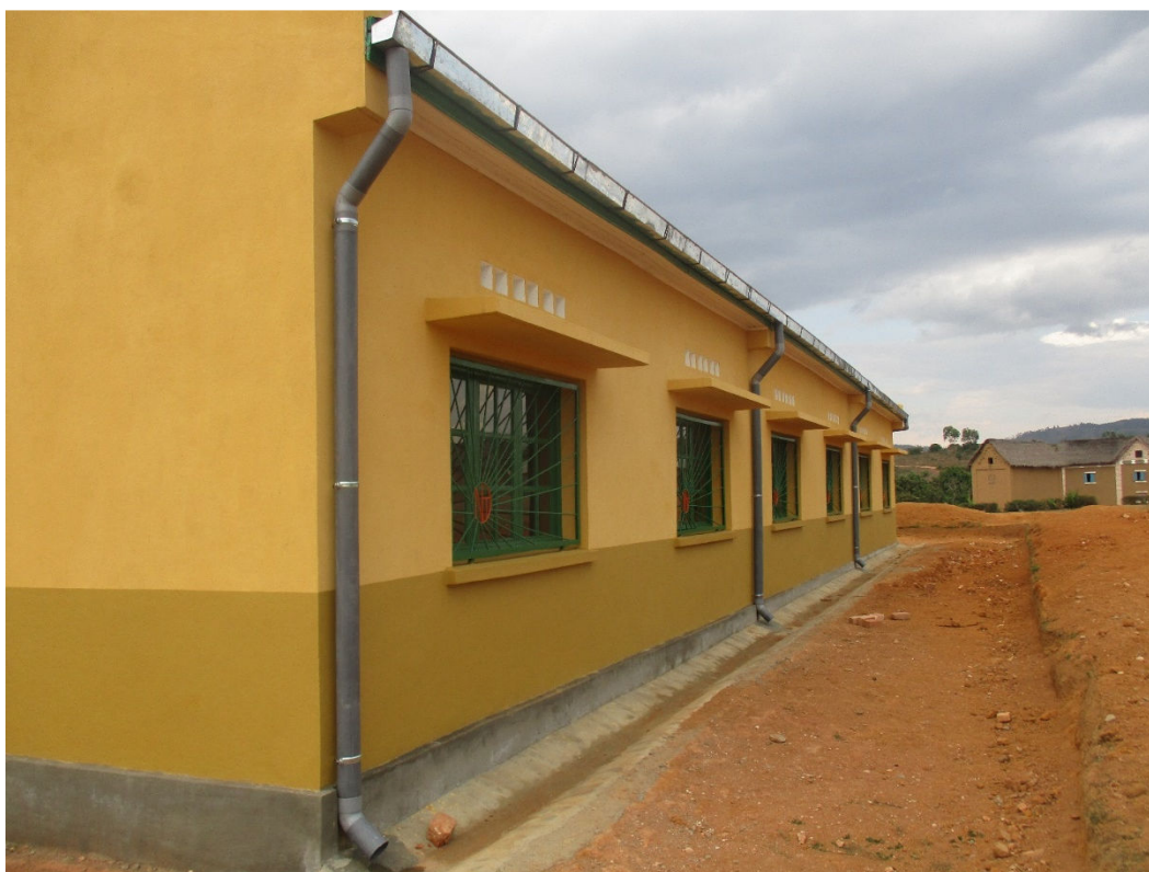
Figure 11: Guttering installed at Tomalaza Secondary School.
