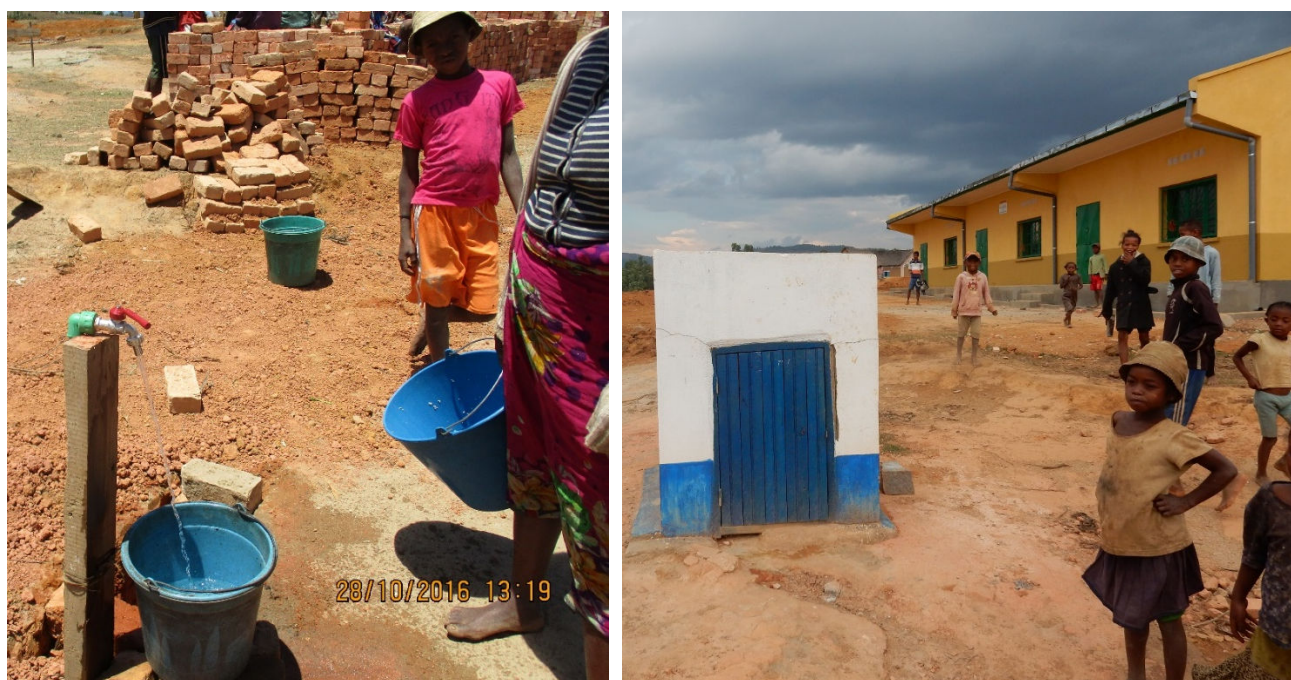
Figure 5: Initial installation of a tap-stand to facilitate building works (left) & protection for the finished tap-stand for use by the school (right).
