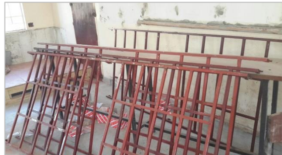
Security bars for the door and windows
