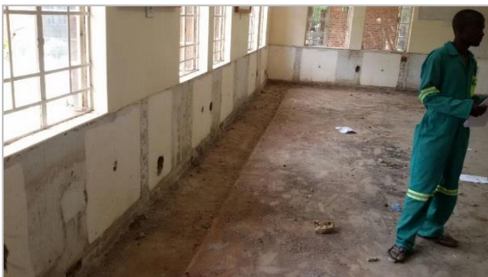
The room is prepared ready for work to begin
