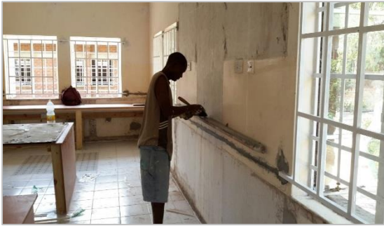
Preparing the walls ready for school colours
