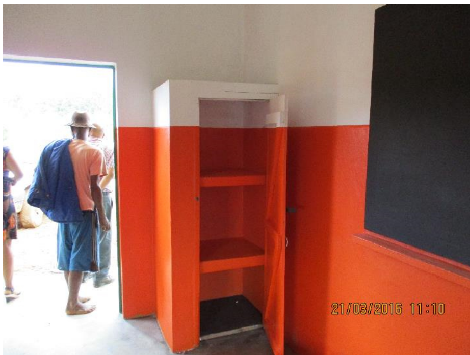
Figure 6: Lockable cupboard in each classroom.
