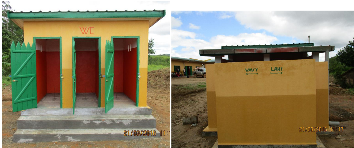
Figure 9: Maromena School sanitation block; latrines & urinals (above & below).
