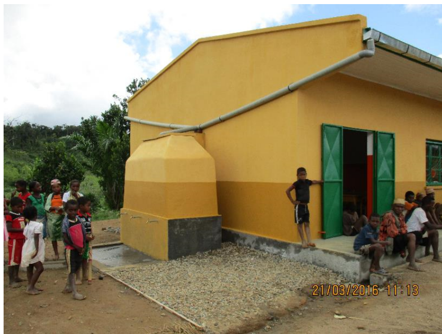
Figure 10: Maromena School impluvium / handwashing point.
