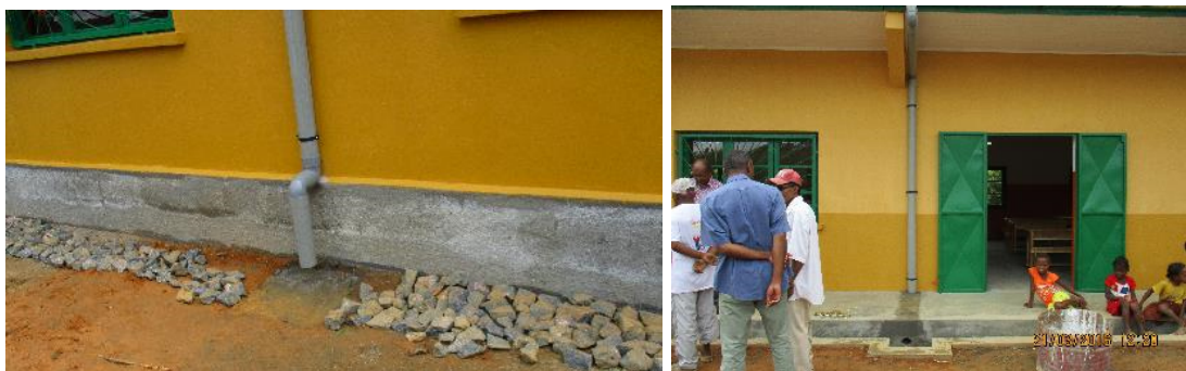
Figure 4: Additional downpipe on the school building.
