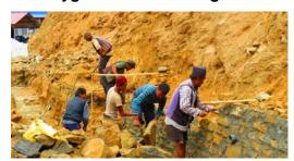
The construction of the new buildings took up most of the outside space, which could have been used for a playground. Therefore, we had to create a wider outside area so that the school could have a playground. In terms of the fencing work, it was felt that retaining walls were a bigger priority, so we used the funds allocated for fencing to construct walls to prevent the soil from eroding away from the school premises when there is heavy rain.
