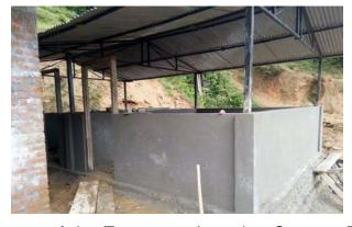
In parallel to the four room brick building, we two-room hollow constructed а concrete building, which is now almost complete apart from installing lightweight walls. We decided to go for hollow concrete blocks instead of stone or brick in order to keep the costs low, as well as to speed up the building process. Hollow concrete blocks are slightly cheaper than bricks as they locally produced and there compromise with quality either. The metal trusses and roof for this building were used from
