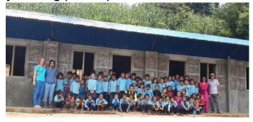
For this building, we followed a standard government model that consists of metal frame with a set of roof trusses supported by metal poles that are fixed to the ground. The walls were made from brick masonry reinforced with horizontal bands.
