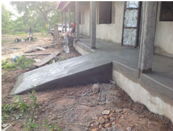
Kabampe Junior High School showing ramps to the veranda and the metal doors awaiting painting.
