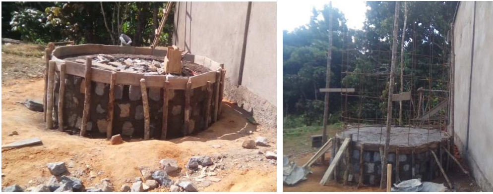
Figure 25: Making the rainwater collection tank using ferro-cement techniques.
