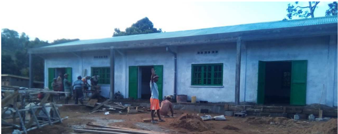
Figure 23: First undercoat of paint (above) & cement flooring (below).
