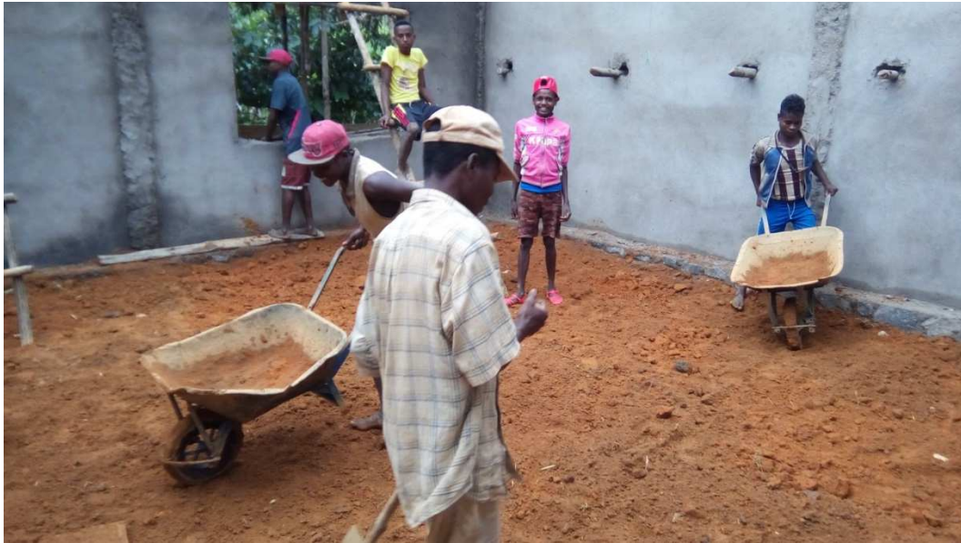
Figure 20: Preparation for the foundations of the cement flooring.
