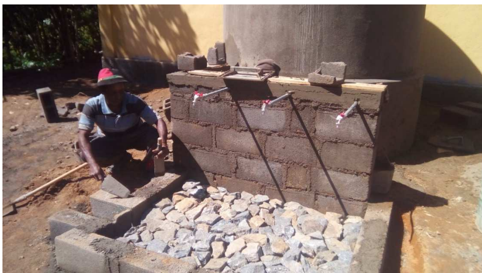
Figure 28: Installing the hand-washing point (above) and finishing touches to the sanitation block (below).
