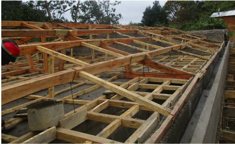
Figure 18: New system of plastered ceilings.
