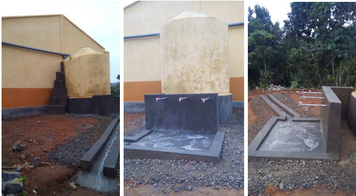
Figure 9: The rainwater catchment system and hand-washing points between the sanitary block and the school.
