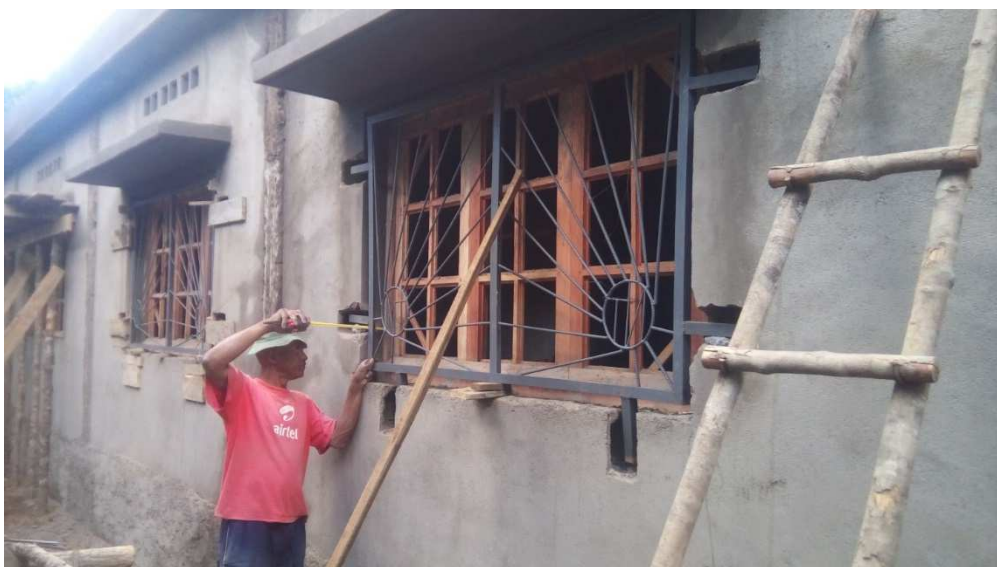
Figure 24: Installing window protection panels.
