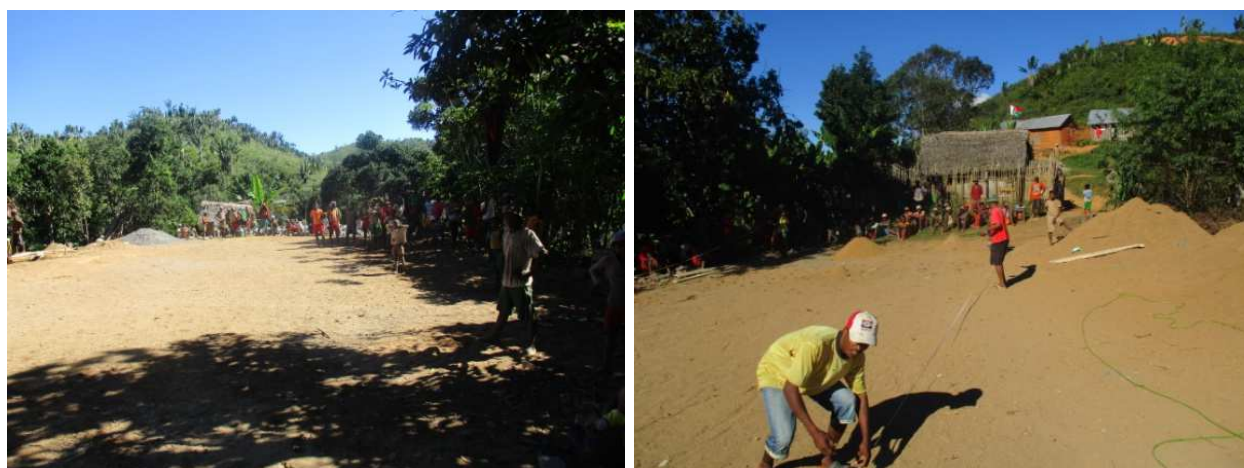
Figure 6: Levelling the land (left) and marking out the ground before starting digging the foundations (right).
