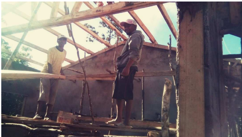
Figure 17: Laying the roof structure.
