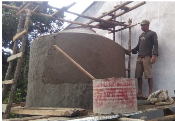
Figure 25: Making the rainwater collection tank using ferro-cement techniques.
