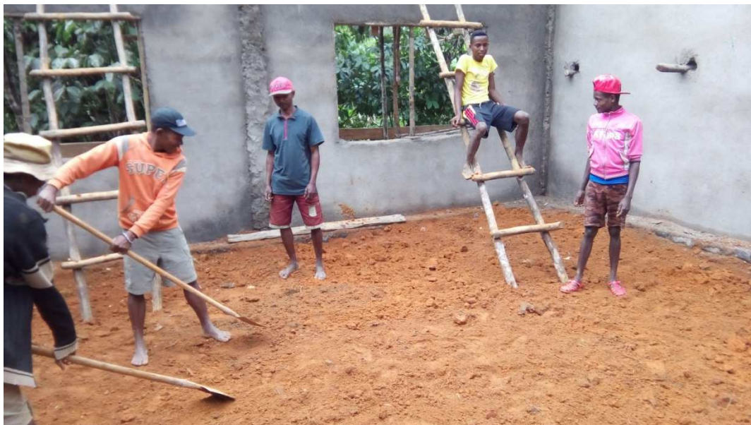
Figure 20: Preparation for the foundations of the cement flooring.
