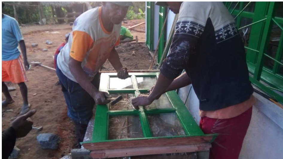
Figure 26: Painting and installing window panes.
