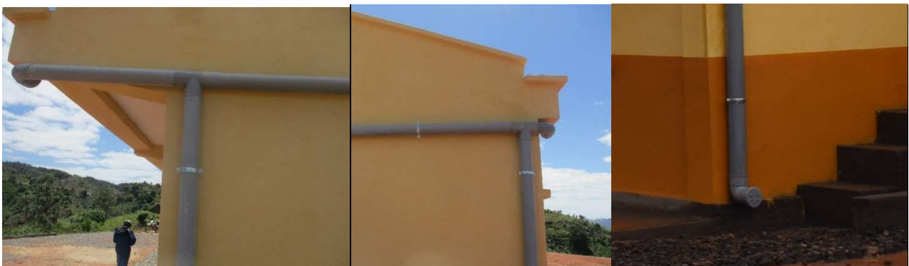
Figure 15: New piping system to divert the first rainwater from entering the tank.
