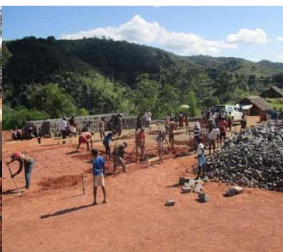
Start of digging the foundations and (right) cement breeze-blocks drying
