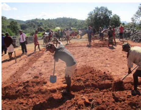
Start of digging the foundations and (right) cement breeze-blocks drying
