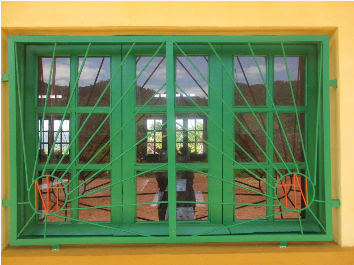
Figure 14: The window protection grill model was changed slightly to strengthen it.
