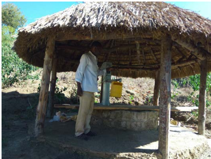
The completed well.
