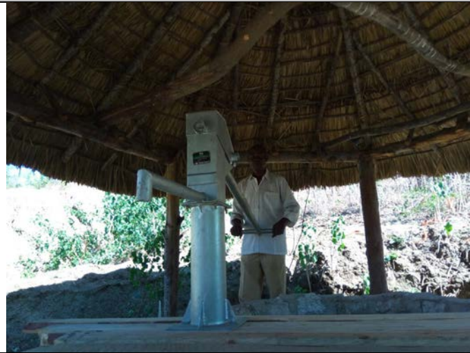
The newly-installed well pump at Jitegemee
