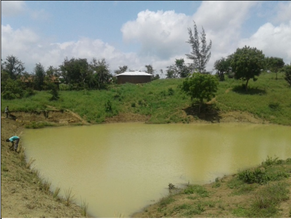
The completed dam at Ufanisi
