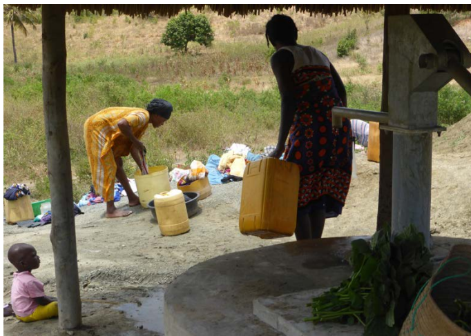
The completed well in use at Dzanikeni
