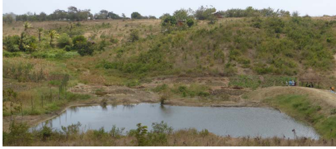
The completed dam at Dzanikeni
