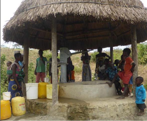
The completed well at Ufanisi
