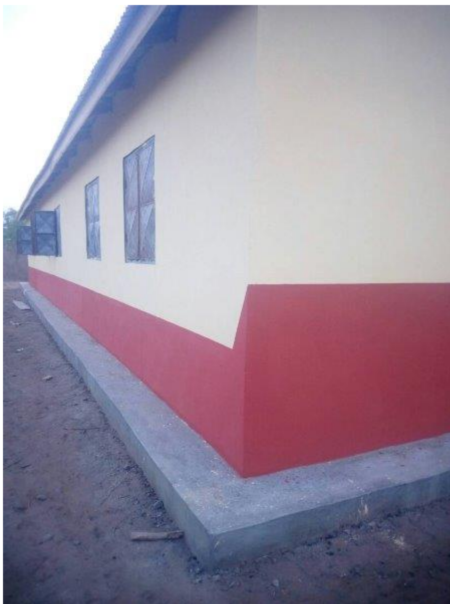
Rear of Koldani School just painted and finished.
