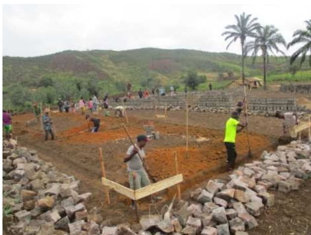
Figure 4: Marking out the foundations
