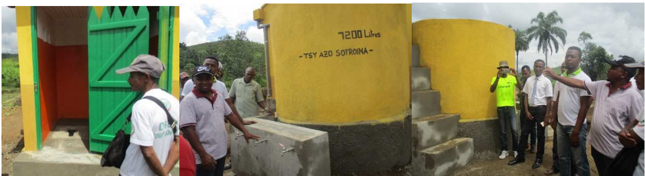
Figure 16: The rainwater catchment system with tap-stands for hand-washing.
