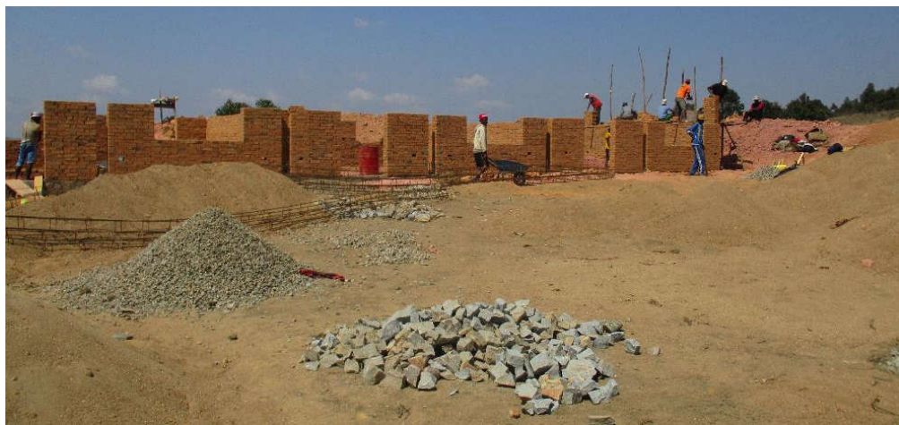
Construction of one classroom building underway.
