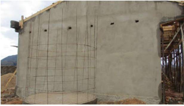
Start of building the frame for the ferrocement impluvium water collection tank.
