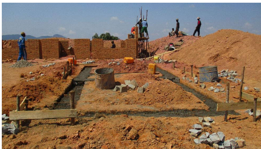
Foundations of the school office building.
