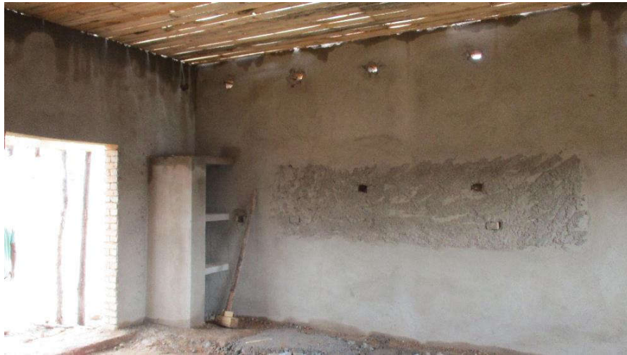
Shelving inside each classroom.
