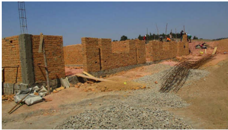
Photos of the school building underway:
