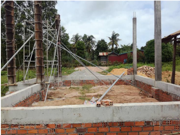
BELOW – photographs showing the phases of construction
