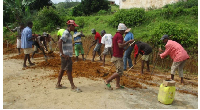
Digging the foundations
