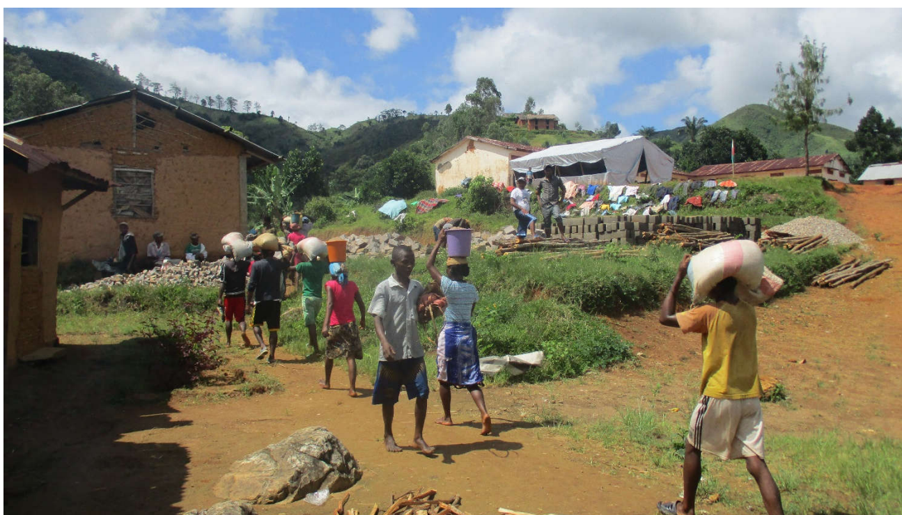
Figure 6: Community contributions to the Ambatofotsy Lycée project: carrying materials to site.
