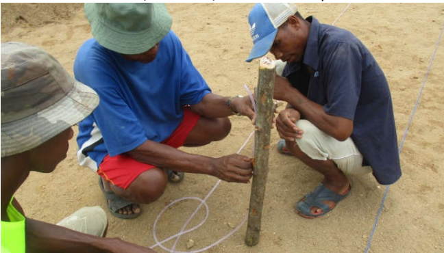
Builders' levelling equipment
