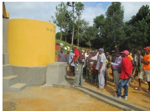
Figure 14: Verification of the implusium rainwater catchment system.
