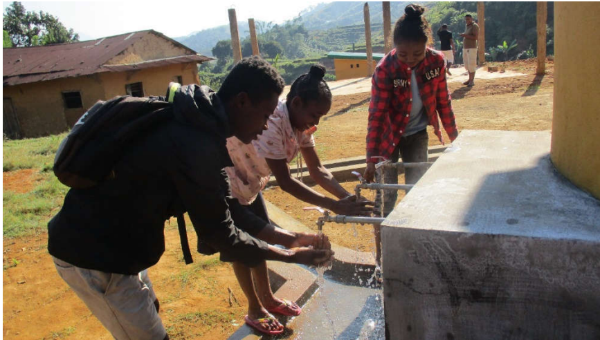
Figure 12: Hand-washing from the rainwater-catchment system at the new school.
