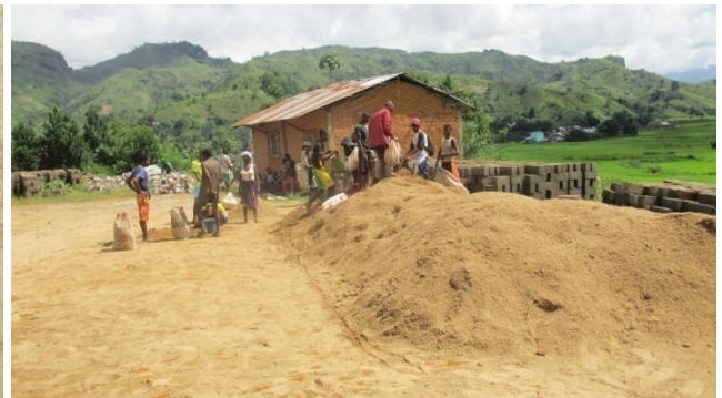
Delivery of sand to the site
