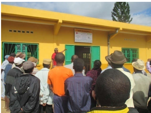
Figure 13: Explanation during the technical verification of works.
