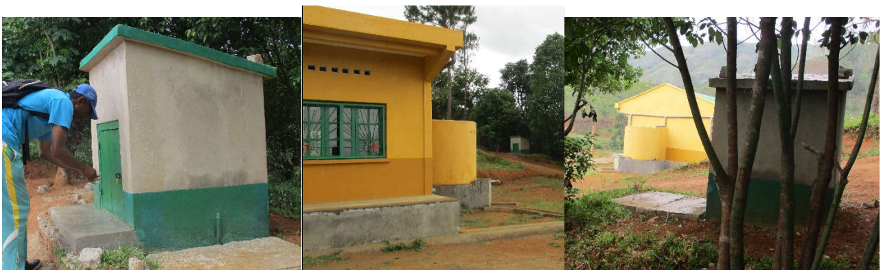
Figure 19: The new tap-stand (lockable for security/to prevent damage) located near to the new school building.
