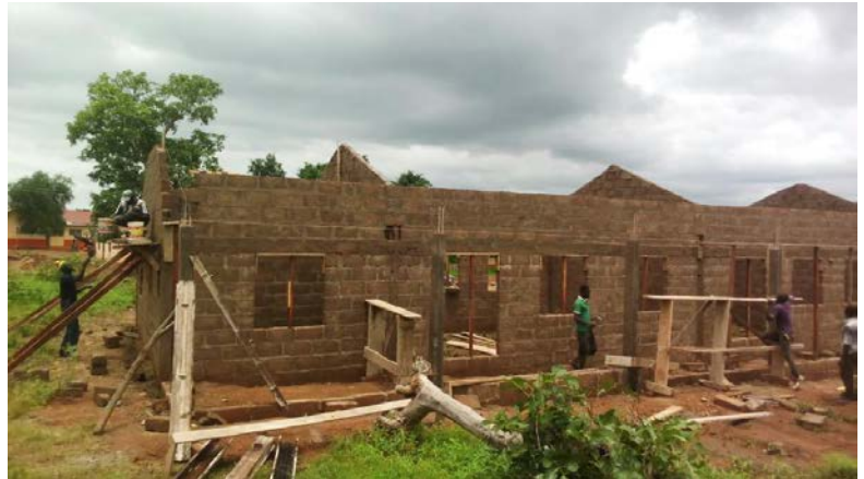
Larabanga JHS under construction June 2011
