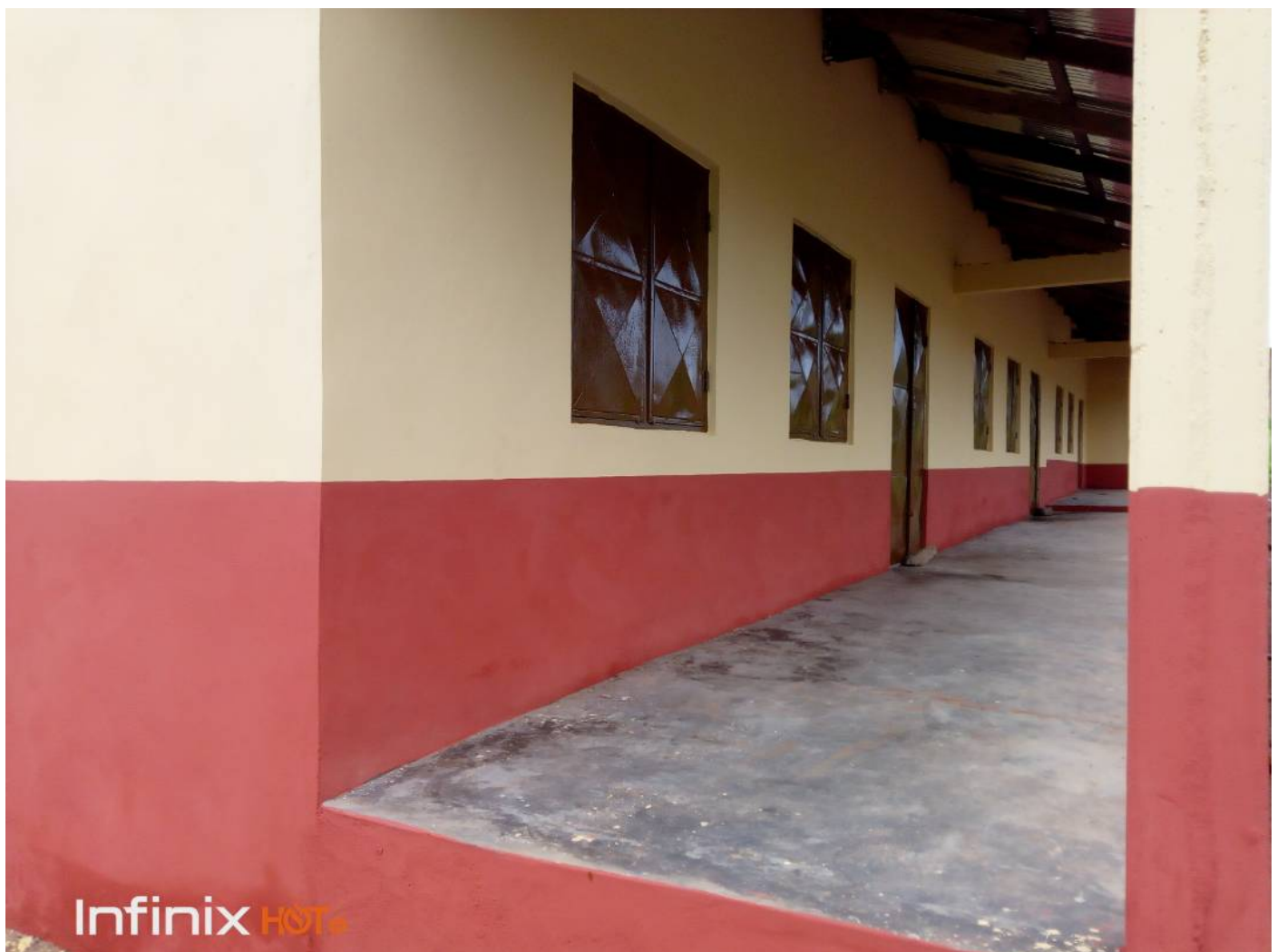
Larabanga JHS completed September 2018
