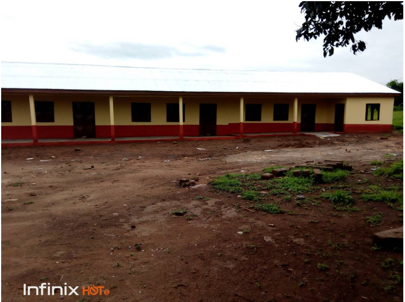
Picture of Larabanga JHS school taken near to completion of 3 Classrooms and storage/teachers room.
